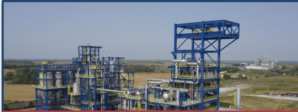
Monolith Olive Creek, NE Methane Pyrolysis H 2 Production
